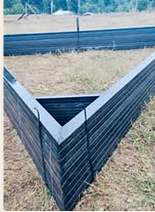
01 Setting out the base
